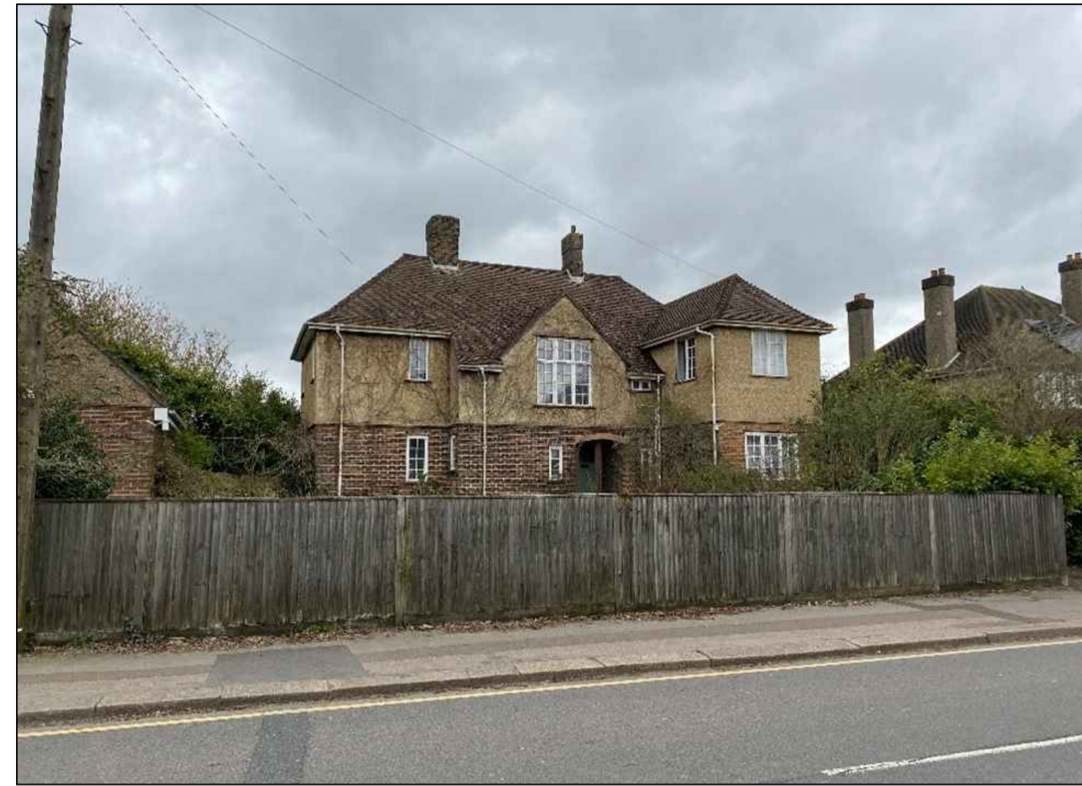
EXISTING FRONT ELEVATION FACING LADBROKE ROAD. THE EXISTING DWELLING PROVIDES NO ARCHITECTURAL INTEREST OR HISTORIC IMPORTANCE.
