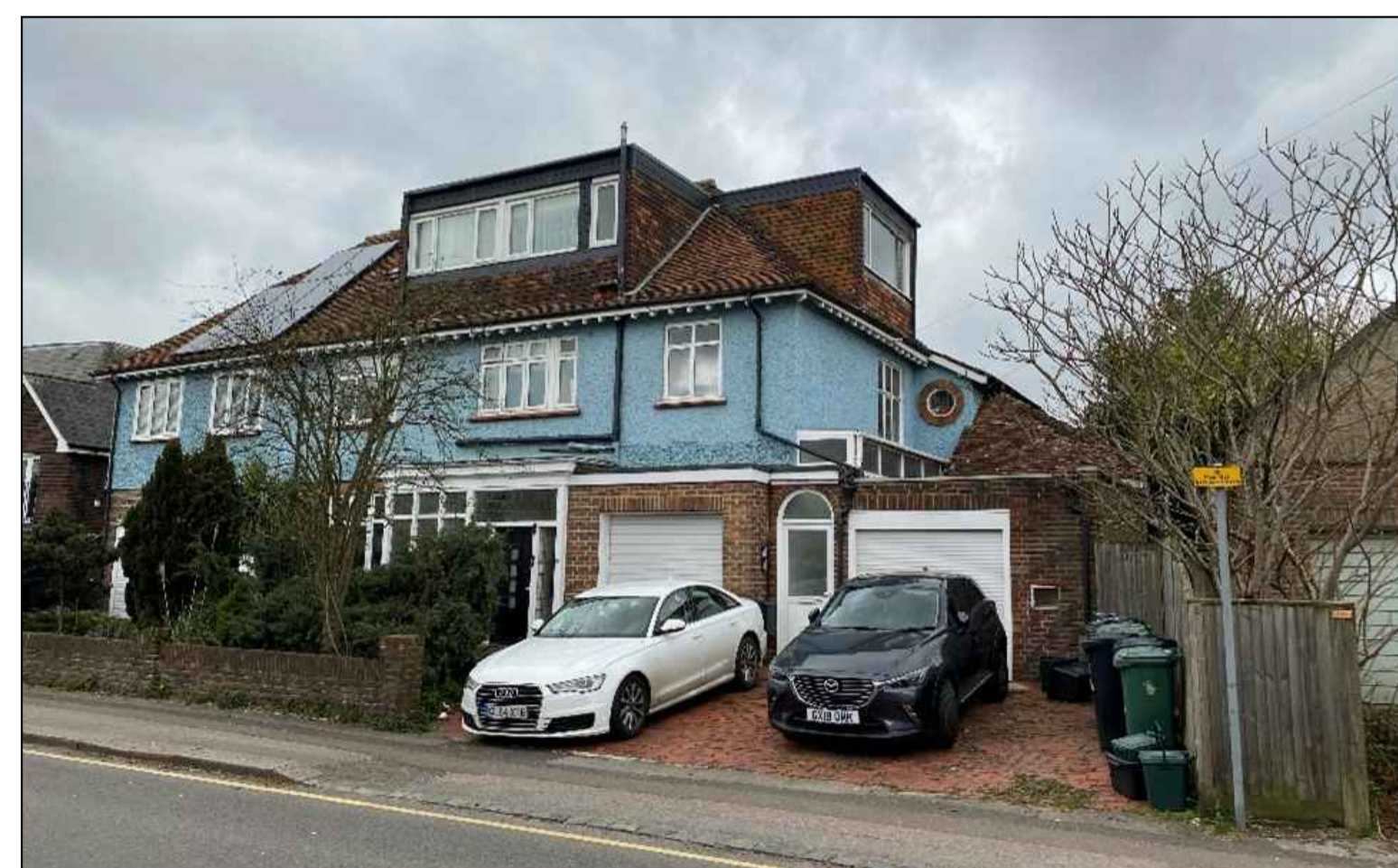
NEIGHBOURING DWELLING WITH SIDE FACING WINDOW. CONSIDERATION HAS BEEN GIVEN WITH A 12 METRE STANDOFF PROVIDED ON A SLOPING ROOF TO RETAIN EXISTING LIGHT.
